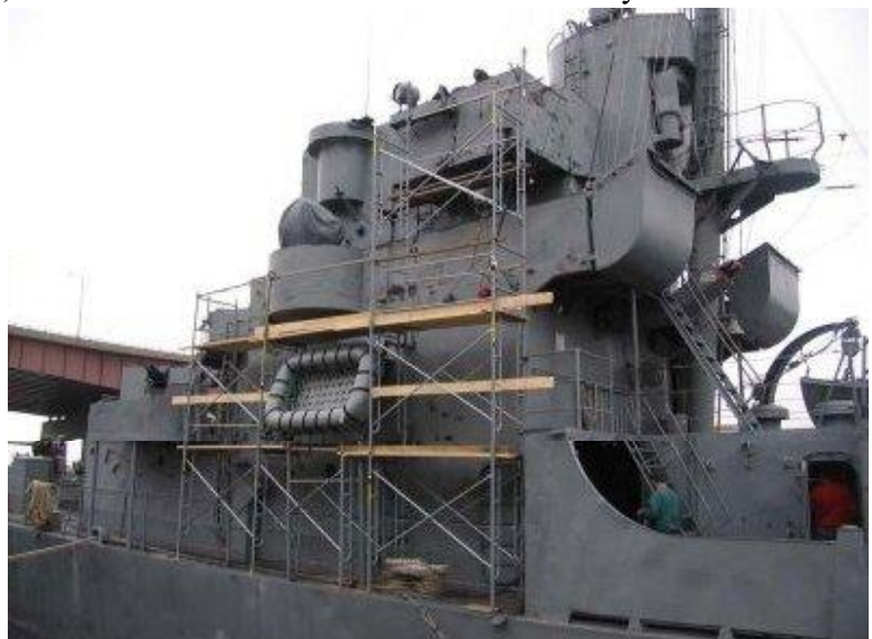
The port side scaffolded and ready for painting.
