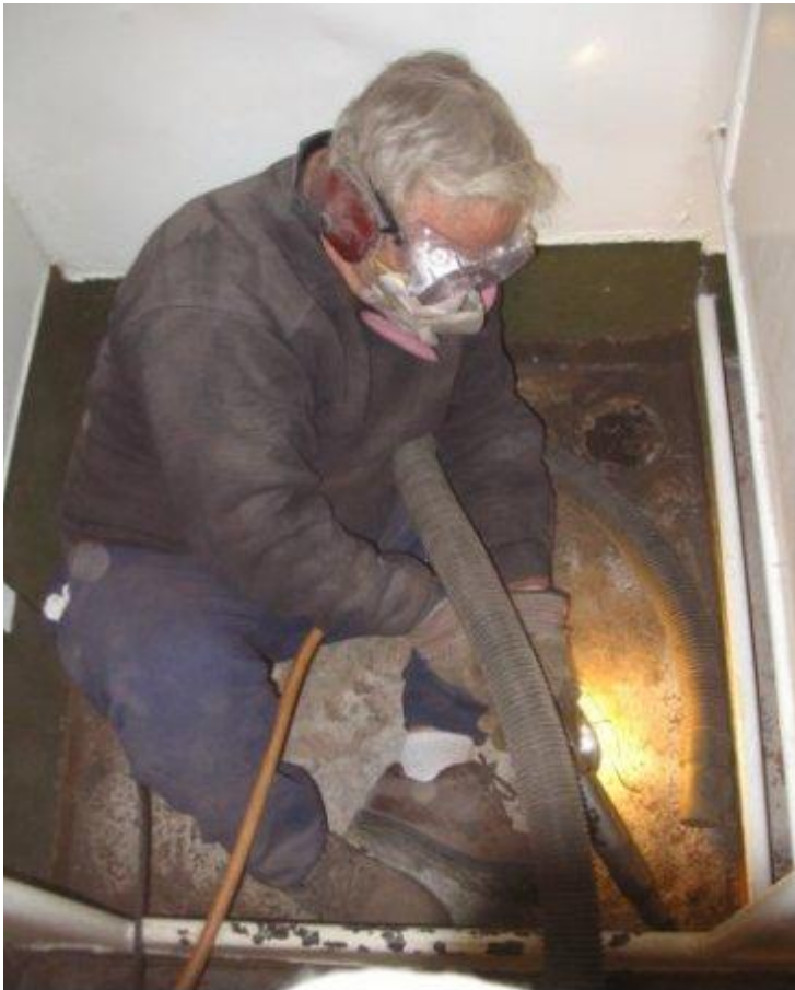
Earl Herchenroder chipping shower stall concrete.
