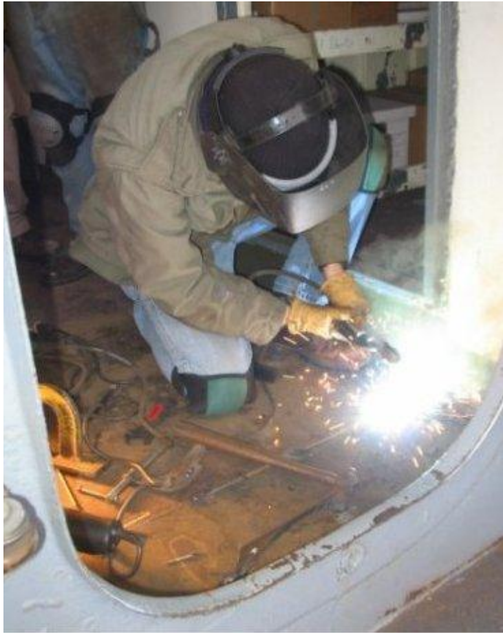
Chuck Teal welds in new passageway deck plate.
