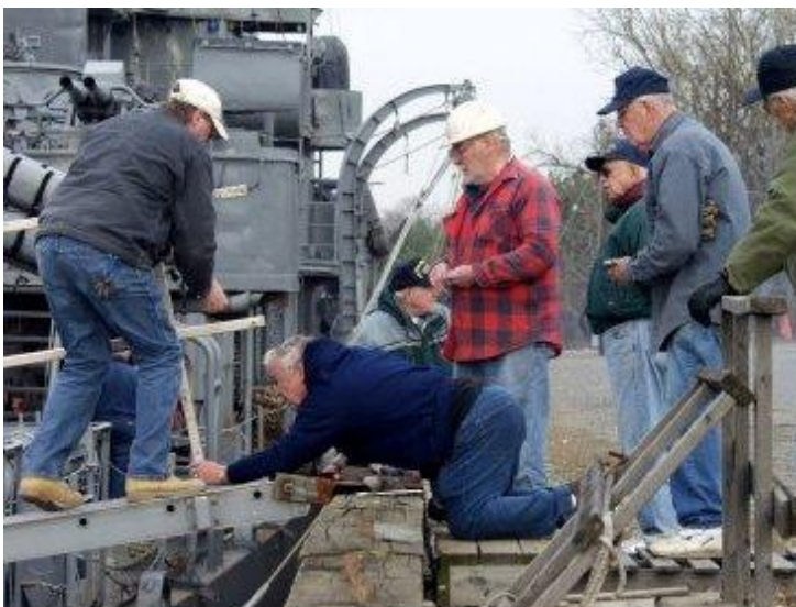
Rigging the gangway handrails after the move.
