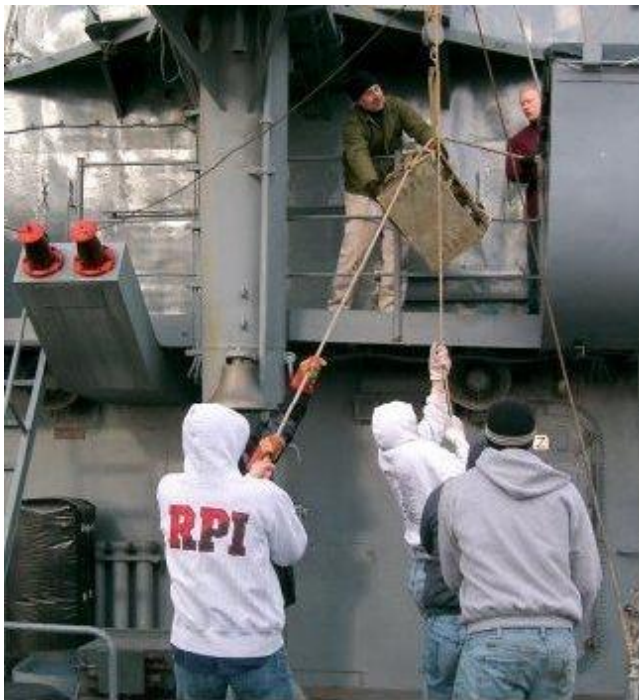
RPI NROTC Cadets hoisting a new radar unit up to the O2 level...
