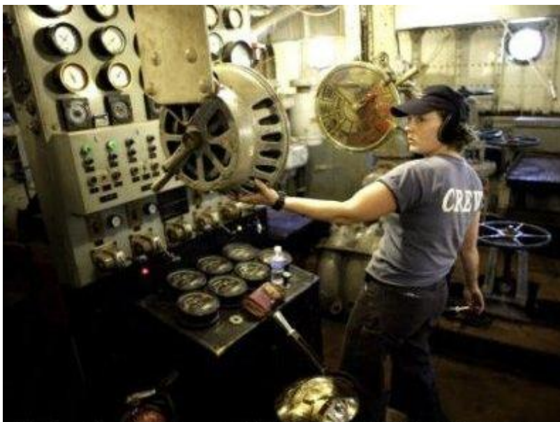
Engineer Jessica answers bells in the HARVEY's engine room.
