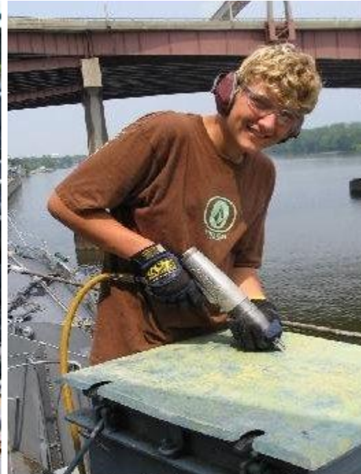
John Kosa is chipping the ammo lockers forward of the pilothouse.
