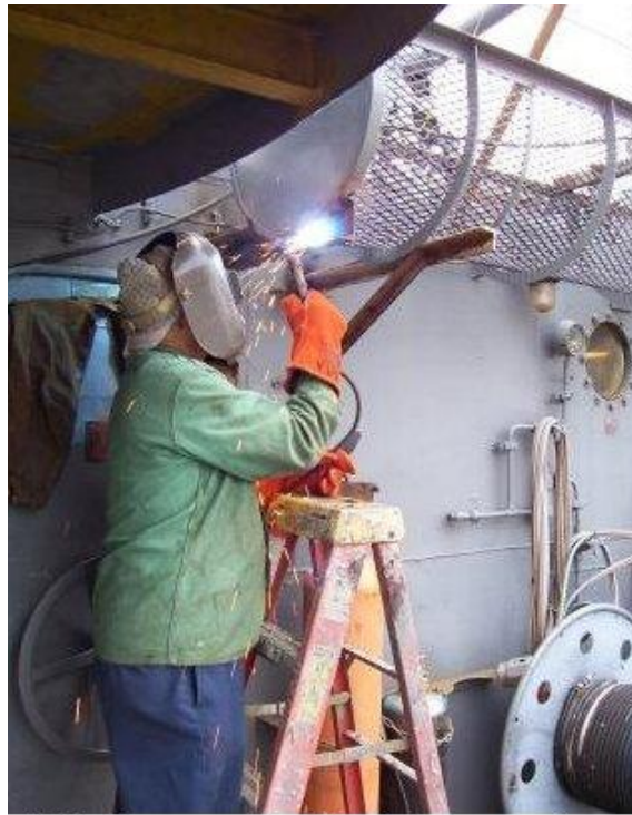
Eighty three year old welder Clark Farnsworth welding up the floater net basket.
