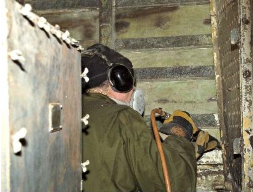
Les Yarbrough scaling in the anchor windlass room.
