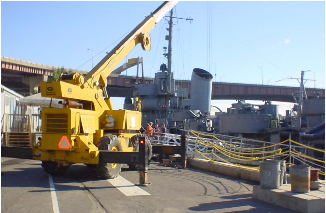
Ready to lift the gangways.
