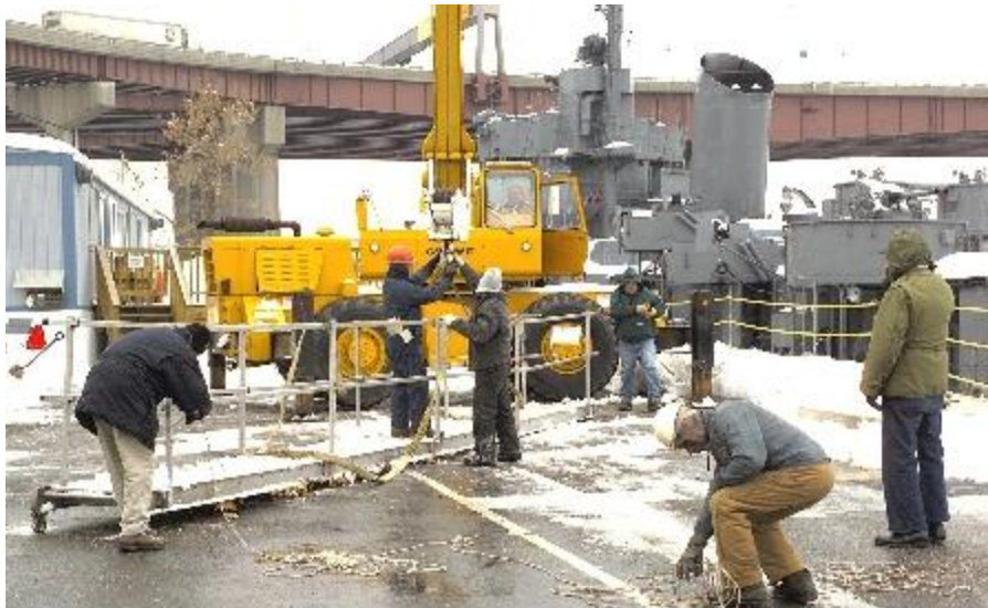
The crew rigs the temporary gangway on December 9th.
