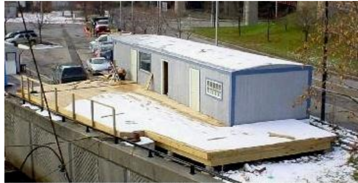
The deck is nearly completed. That white stuff is November snow.
