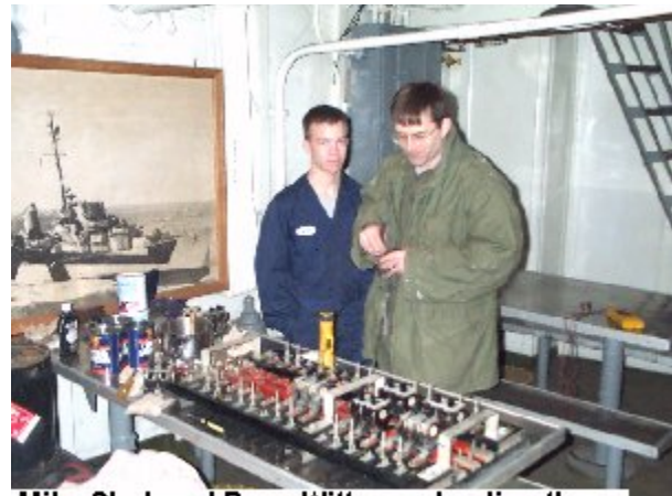
Mike Clark and Barry Witte overhauling the new Galley Breaker Panel.
