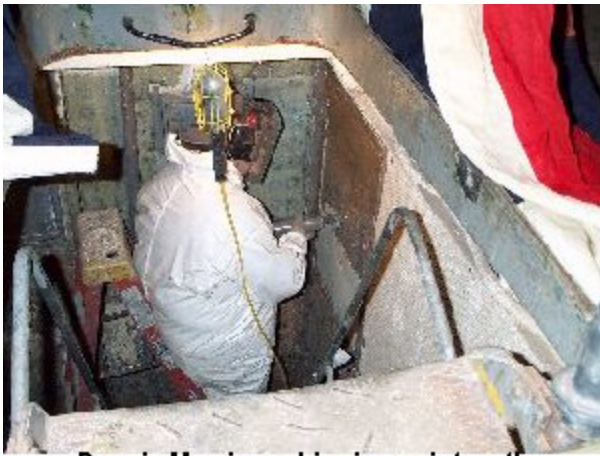
Dennis Morrissey chipping paint on the Reefer Deck
