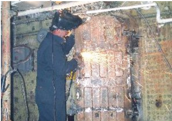
Remember the old shipyard slogan, "If you want Kill time try Working it to Death." Tim Brenner working on the Watertight Door.
