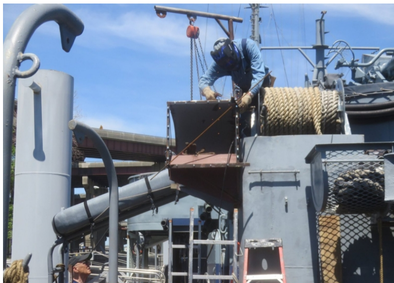
Work continues on the aft supply vent fan intake.
