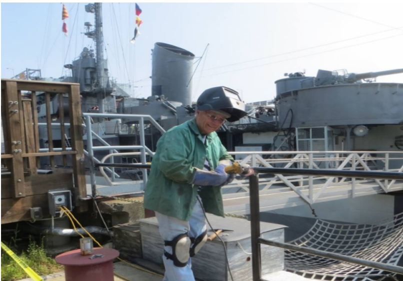
The shipfitters are making great progress on the seawall safety railing.
