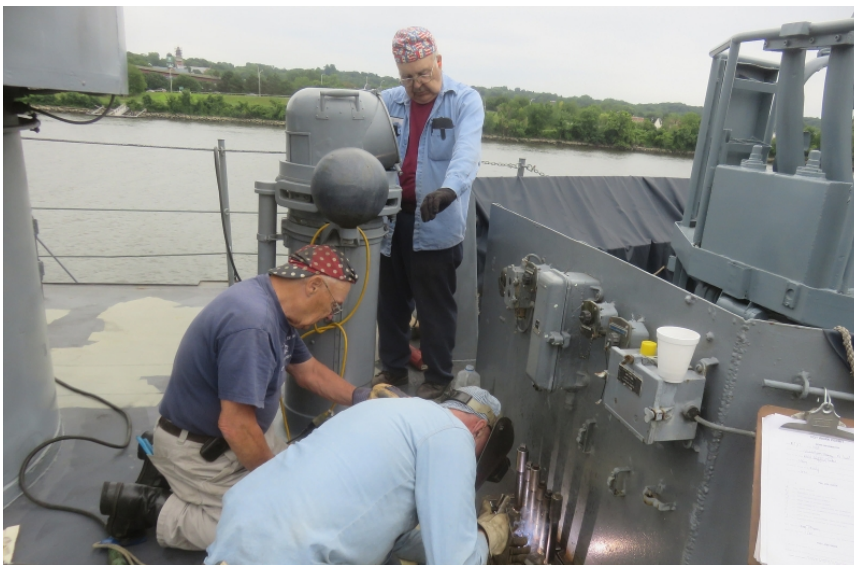
Replacing the electrical stuffing tubes at the secondary conning station.
