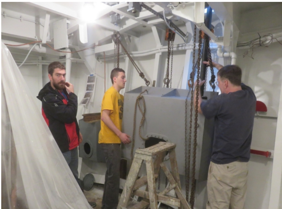
Installing the smoke generator tank.
