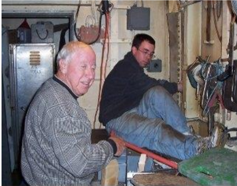
Don Bean and Paul Suzdak working the expansion joint.
