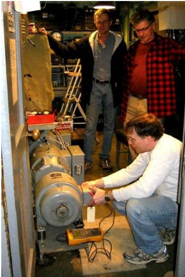
Barry Witte checks out the TBL motor generator as Mike Wyles and Joe Breyer stand by.
