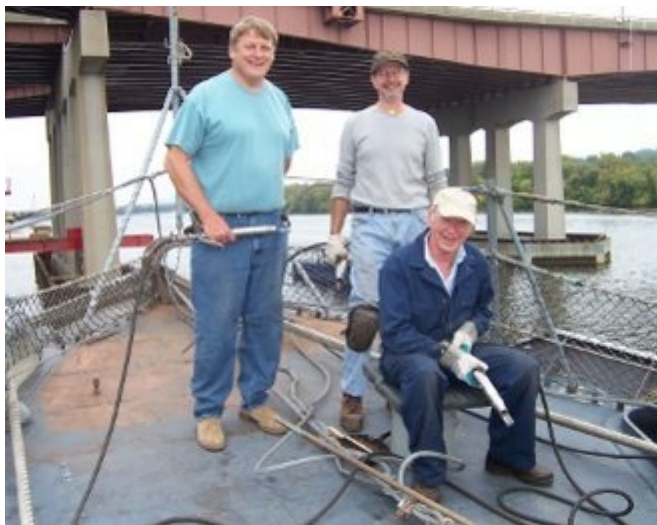
Chippers John Yokum, Ron Prest and Ron Mazure scaling the foredeck.
