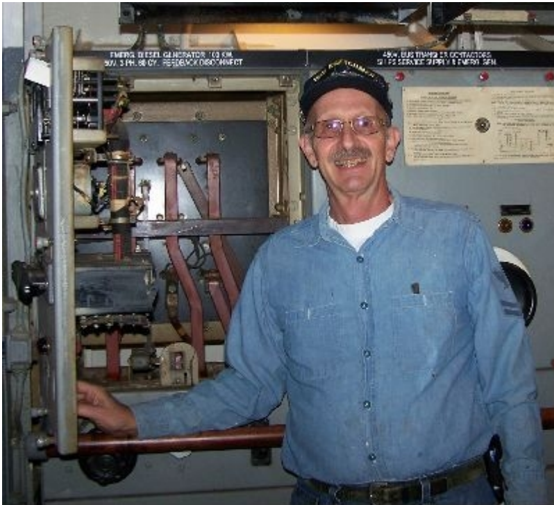
Peter Gamwell cleaning the emergency diesel switchboard.
