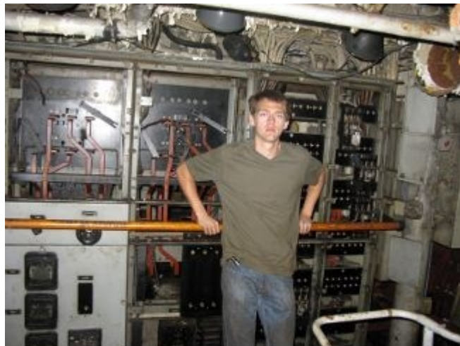
Brian Goodman stripping the switchboard.
