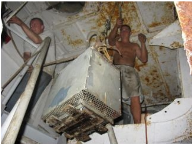
Chris Dennis and Mike Malone hoisting out a transformer.
