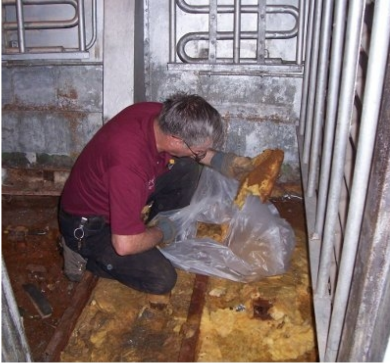
Sheedy bagging wet insulation.
