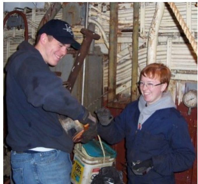
RPI NROTC Midshipmen Ray Osborne and Liz Church reassembling fire and bilge valves.
