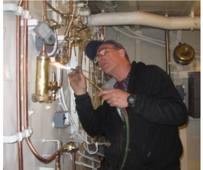
Gary Sheedy working on refrigeration piping on the reefer deck.
