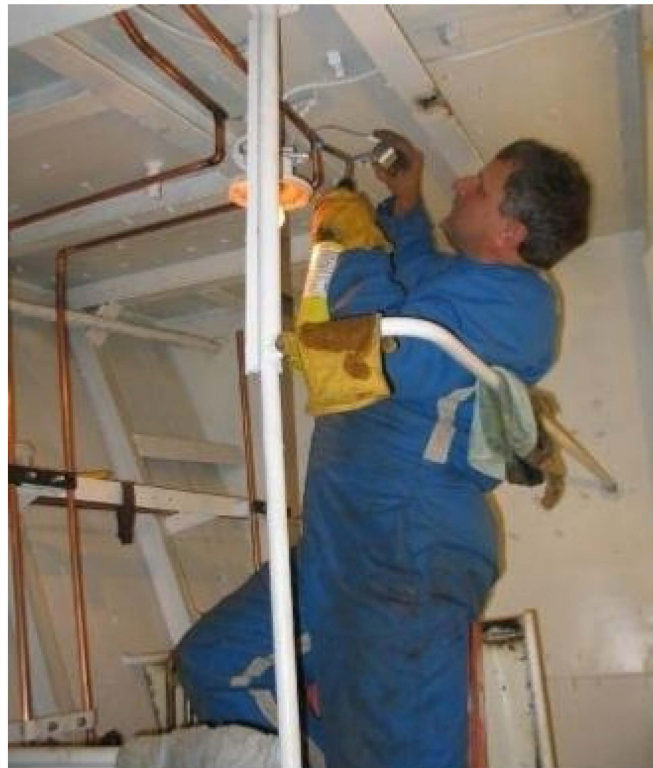
Joe Parker plumbing up the showers in the Forward Crew's head.
