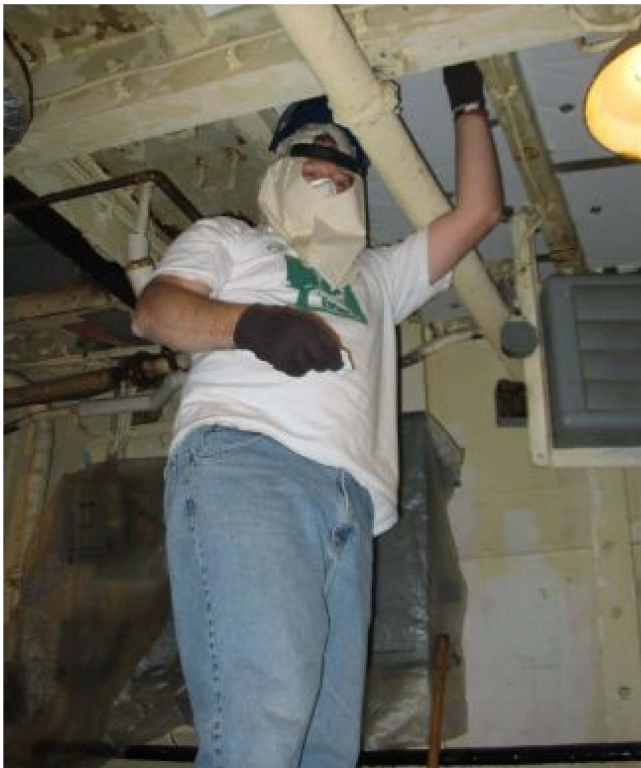
Scott McFadden repairing fiberglass insulation in the aft motor room.
