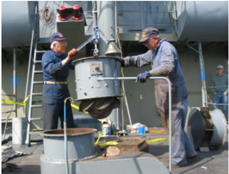
Guy Huse and Butch Warrender pulling apart the galley exhaust fan.
