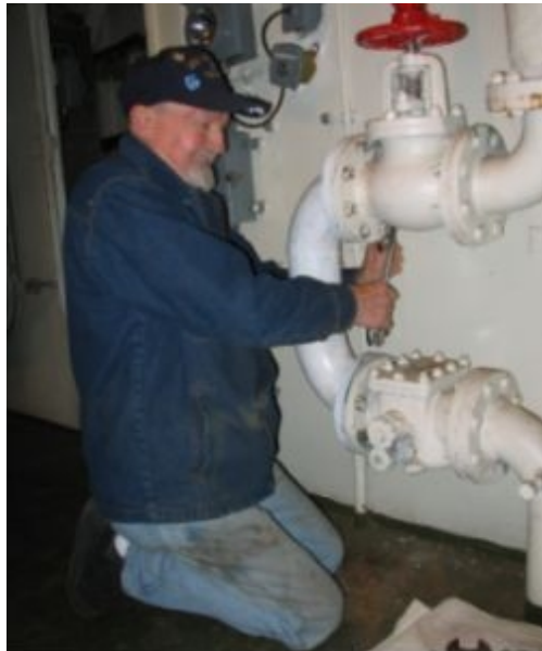
Ed Vallad repairing the firemain in the DE Museum space.
