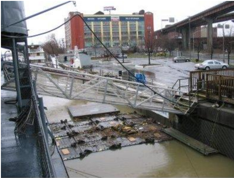
Just after moving the river rose over six feet. The ship end of the gangway should be lower than shore.
