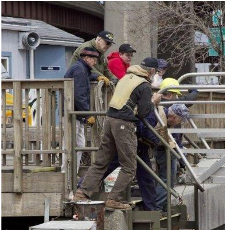
The shore crew manhandles the gangway into place.
