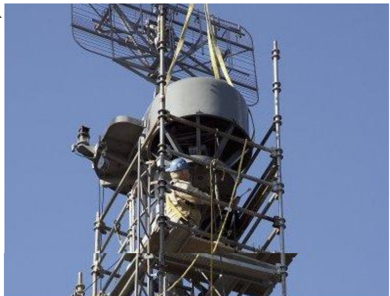
Doug bolts the dome to the platform.
