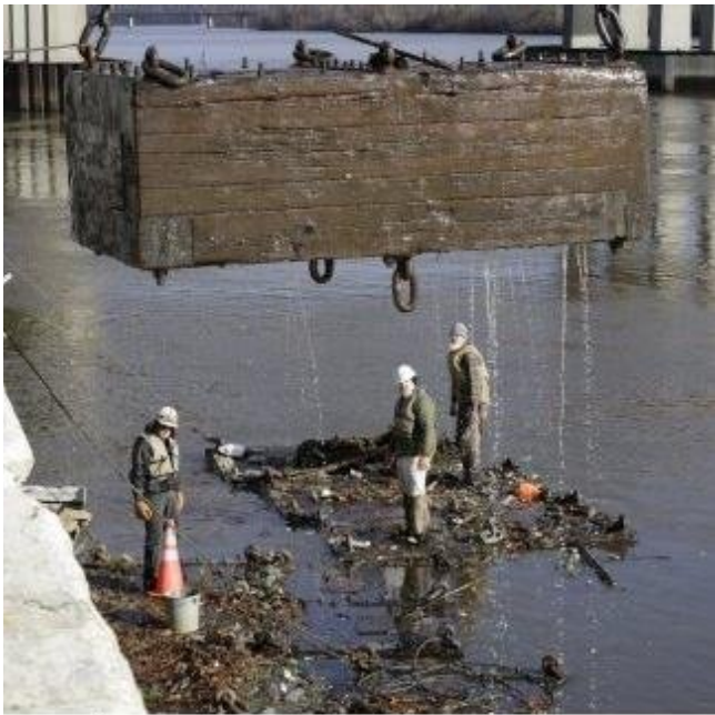
Camels are rigged by the river crew....
