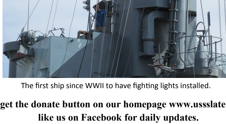
The first ship since WWII to have fighting lights installed.
