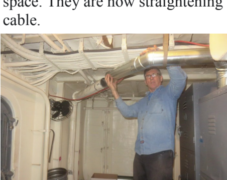
Gary Sheedy fabricating missing duct-work in the aft berthing space.
