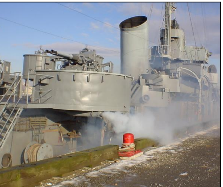
2002, the first start up of the emergency diesel generator.
