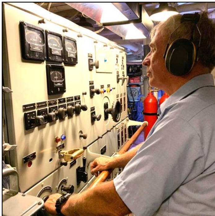
Gary Sheedy on switchboard watch on the way to the shipyard.
