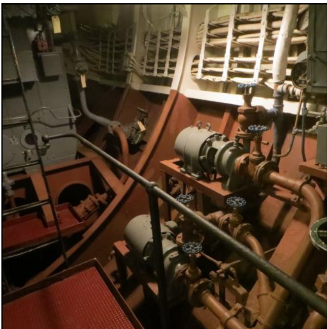
A look at the fresh water pumps after restoration.
