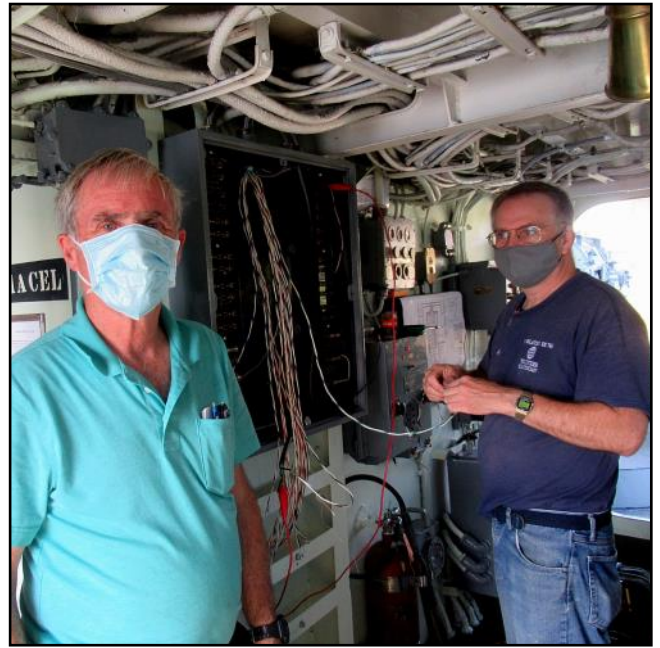
Gary and Barry, wiring in the recognition light panel.
