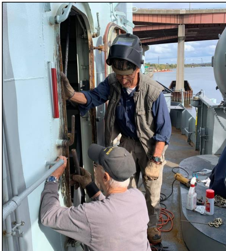
Tim Benner and Super Dave working on those watertight doors.
