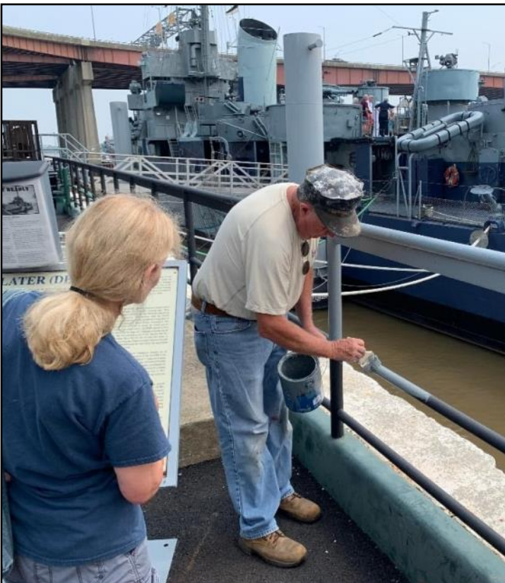
Dennis completed repainting the seawall railing, to make Shanna happy.
