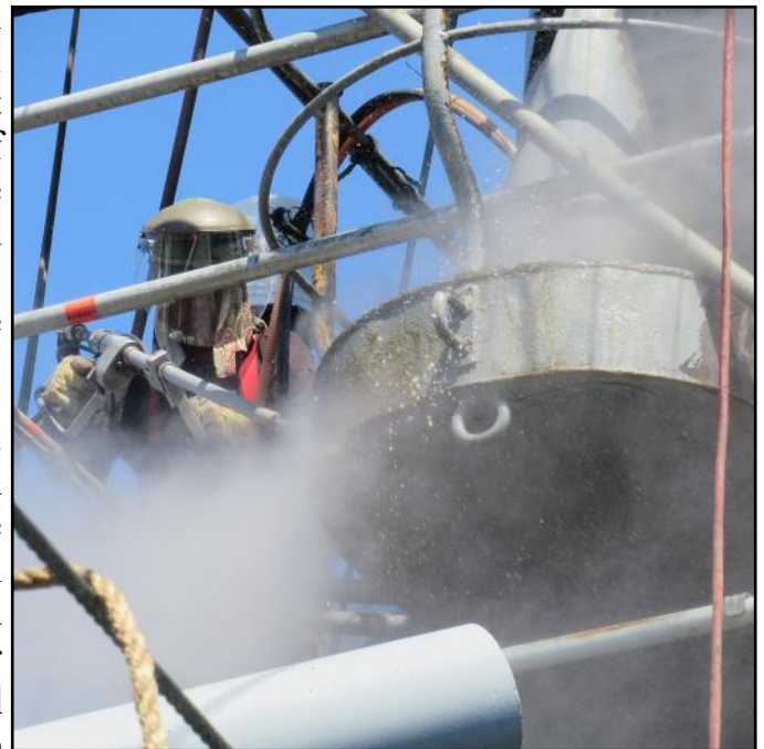
Hydro blasting the mast.
