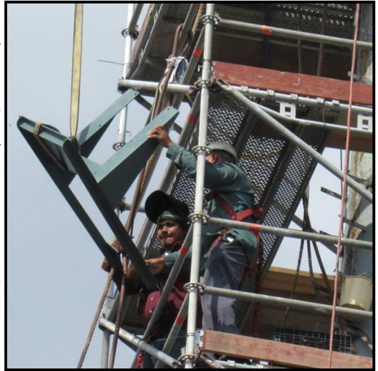
Hauling the bullhorn bracket up.
