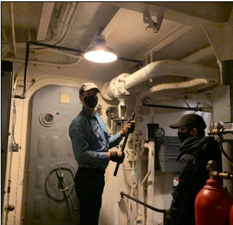
Father and Son team Burgeois replacing steam lines.
