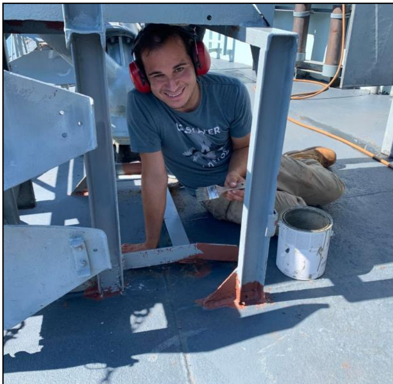
Thomas priming under the depth charge rack.
