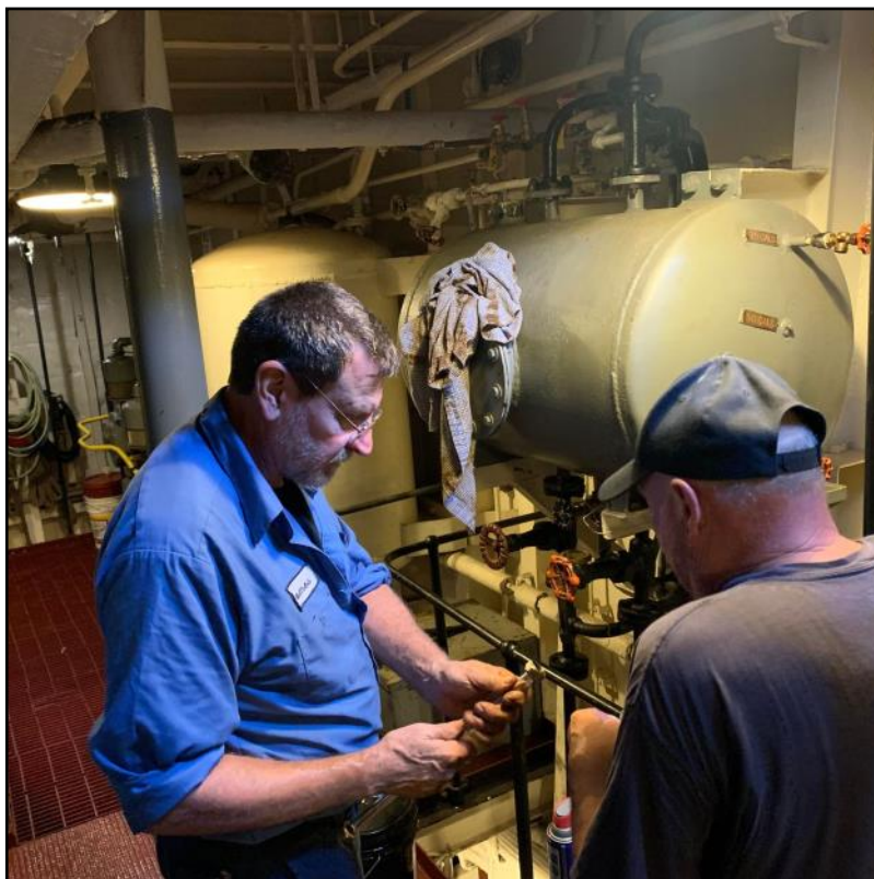
Jim and Mike in the engine room.
