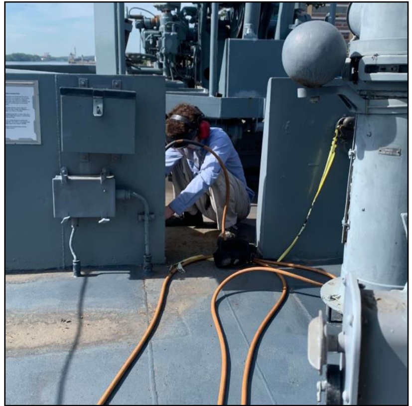
Charles working on chipping paint around the aft 40 mm.
