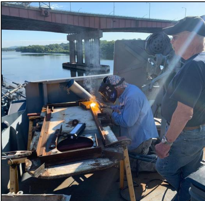
Doug and Super Dave are still working on the watertight doors.
