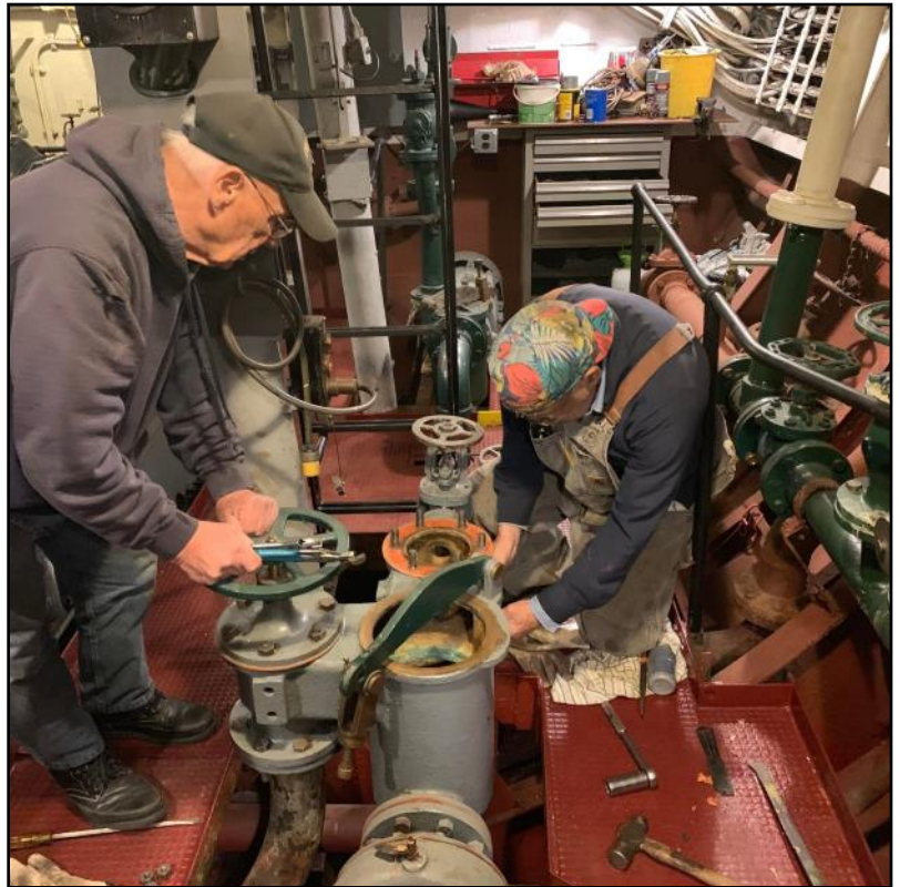
Our volunteers keep a close watch on the bilges for any sign of leakage.
