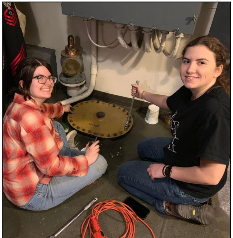
Our RPI Midshipmen doing our annual tank and void checks.
